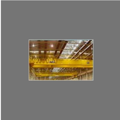
EOT Cranes Modernization
