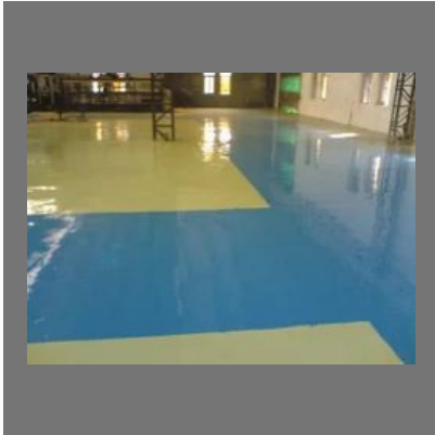
Epoxy Industrial Flooring
