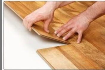
Interiors Flooring Work
