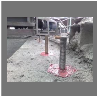
Chemical Anchoring Service
