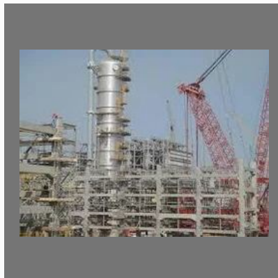
Chemical Plant Construction
