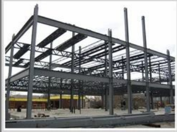
Structural Steel Fabrication and Erection
