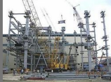
Chemical Plant Construction
