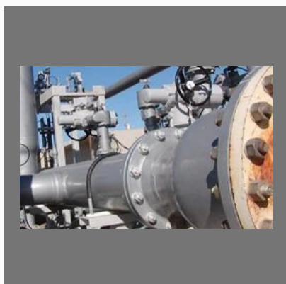
CS And SS Piping Fabrication And Erection
