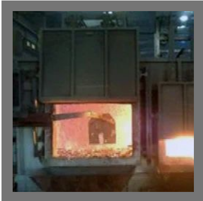
Melting Plant Furnace
