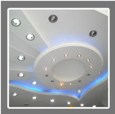
Thermocol Ceiling Works
