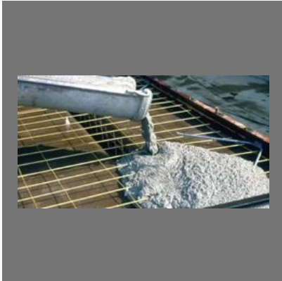
Ready Mix Cement
