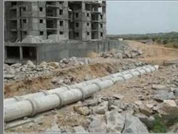
Pipe Laying Work
