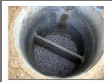
Rainwater Harvesting System Construction
