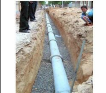
Sewer Line Construction
