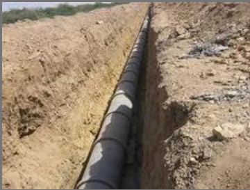
Sewer Pipeline Work
