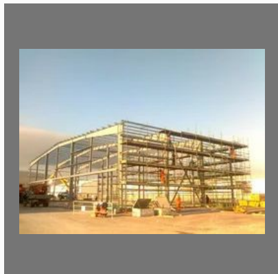
Industrial Construction Projects
