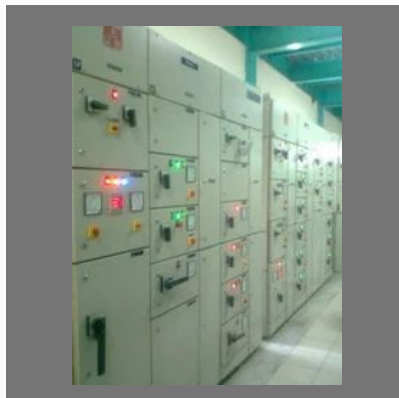
Control & Relay Panel Erections
