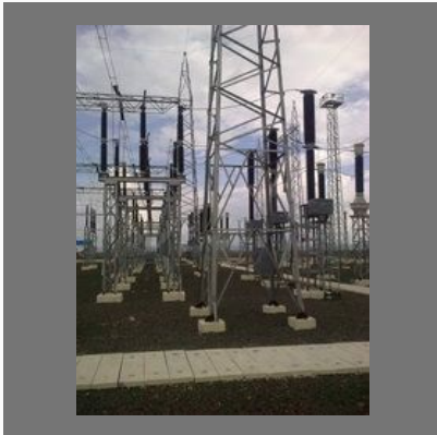
EHV Substations Erection & Commissioning
