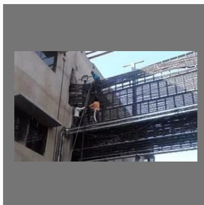
Cable Installation Services
