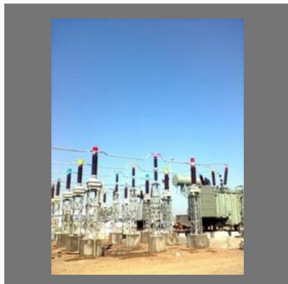
Erection And Commissioning Of Power Transformers
