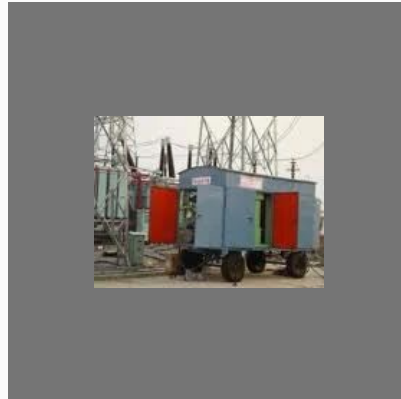
Transformer Oil Filtration Services
