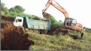
Earthwork Excavation Contracting Service
