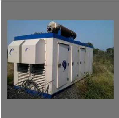
Ashok Leyland Generator Repairing Services
