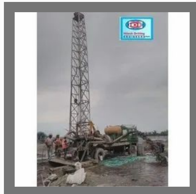
Borewell Installation Service
