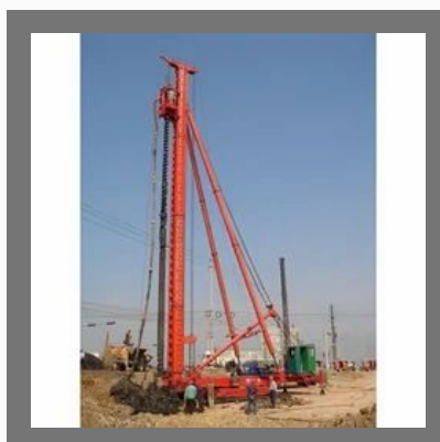
Drilling Pile Foundation Service
