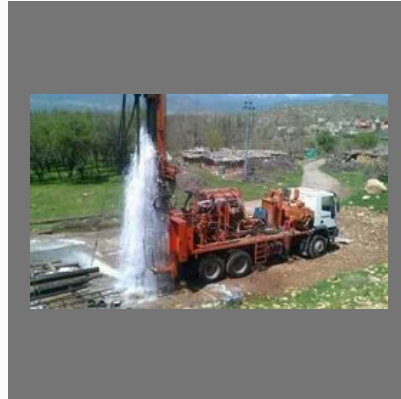
Commercial Borewell Drilling Services
