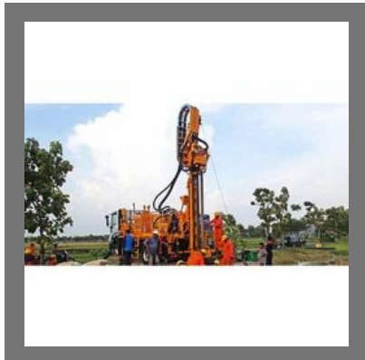
Geothermal Well Drilling Service
