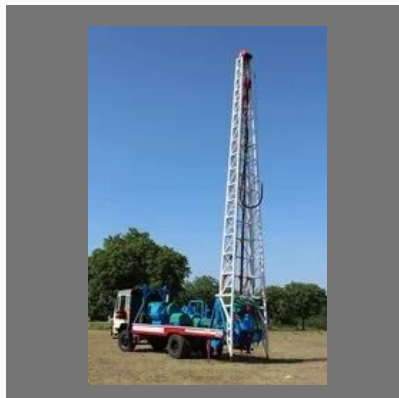
Tube Well Drilling Works
