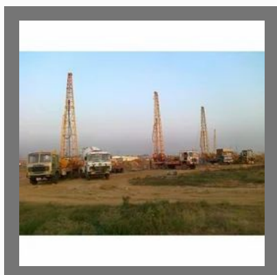
Pile Foundation Services
