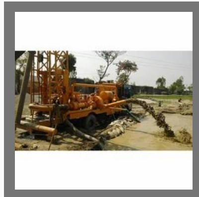
Borewell Drilling Services
