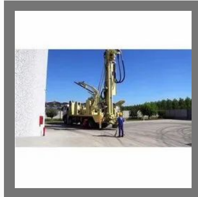
Tubewell Drilling Services
