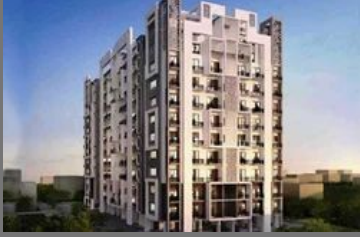
Mandakini Project Building Construction
