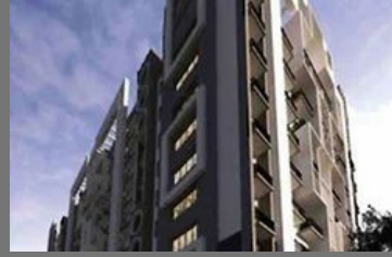
Avyakta Project Building Construction
