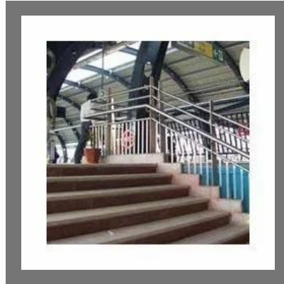
Steel Railing Metro
