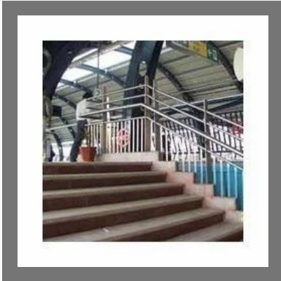
Steel Railing Metro
