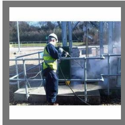
ETP Maintenance Service
