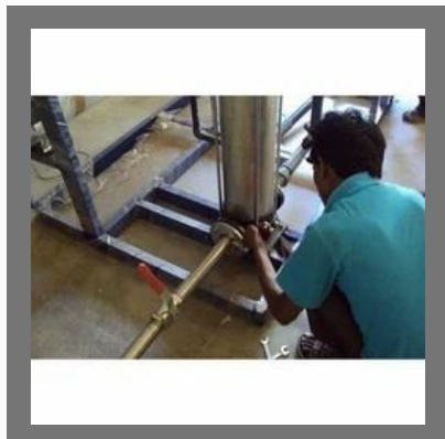
Water Treatment Plant Repairing Service
