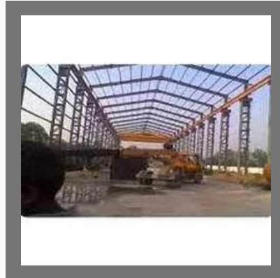
Roofing Turnkey Project
