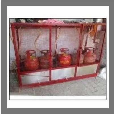
LPG Manifold System
