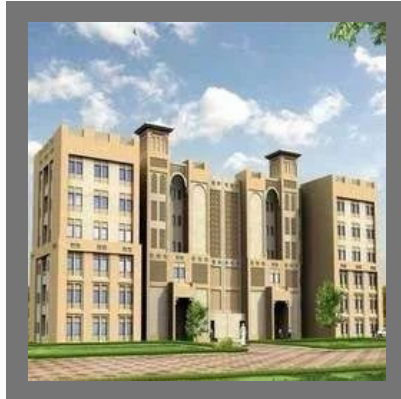
Flats Construction Services
