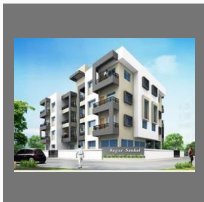
Sagar Sankul Residential Construction
