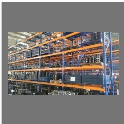
Selective Pallet Racking
