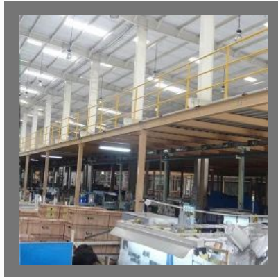
Warehouse Mezzanine Floor
