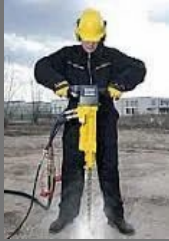
Hydraulic Rock Drills with Rock Splitter
