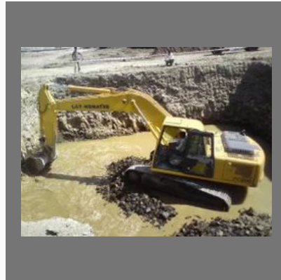
Excavation of soft rock
