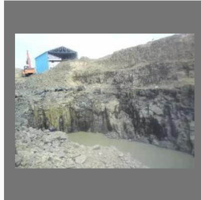
Deep Excavation Service
