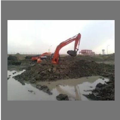
Excavation of all types soil
