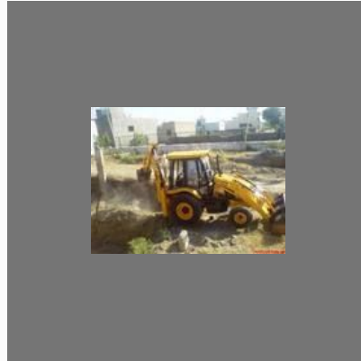
Mico Bosch Hanger Construction Service
