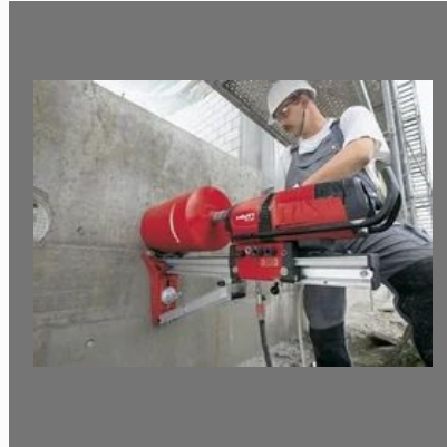
RCC Core Cutting
