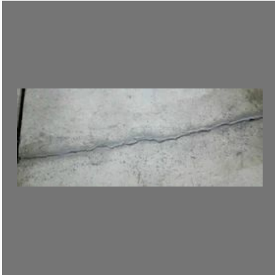
Crack Repair Mortar
