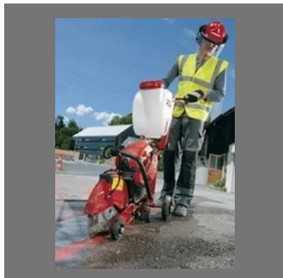
RCC Floor Cutting
