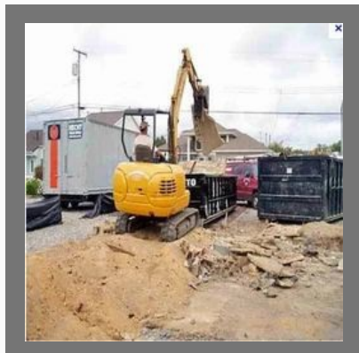
Industrial Demolition Service
