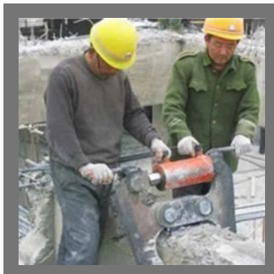
Demolition Concrete Services
