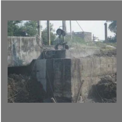
Diamond Wire Sawing Services
