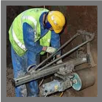
Concrete Core Cutting
