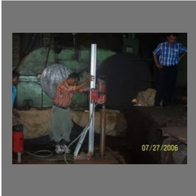
Core Drilling Services
