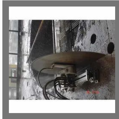
RCC Cutting Services
