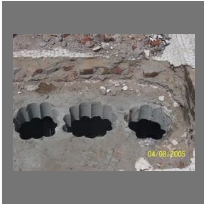
Core Drilling Services
