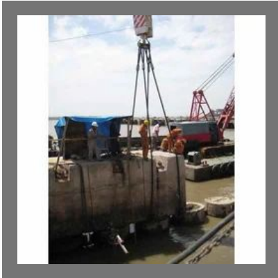
Underwater Concrete Cutting Services
