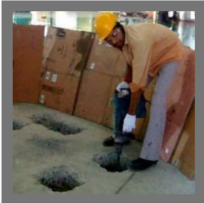
Breaking Concrete Services
