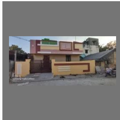
Individual House Construction Service
