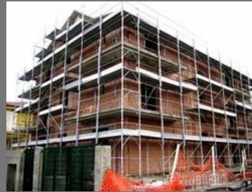
Building Construction Project
