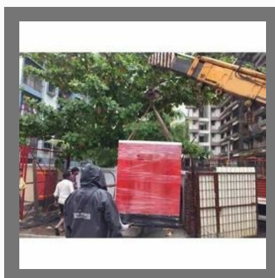
Generator Installation Services
