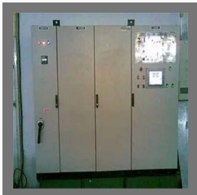
Textile Blow Room Machine
