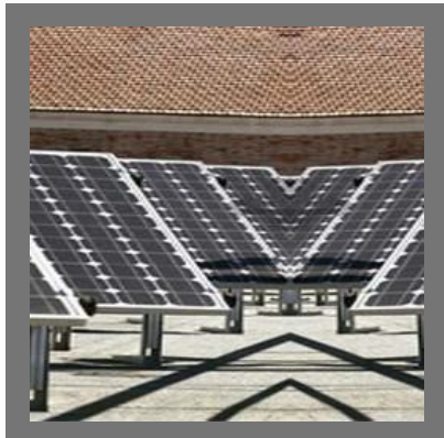
Dismantling & Re-erecting Services
