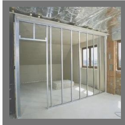
Gypsum Drywall Partitions
