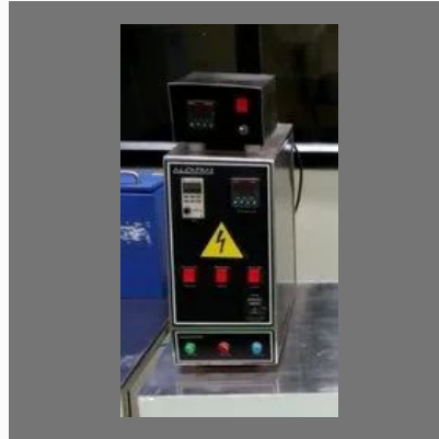
Ss Control Panel
