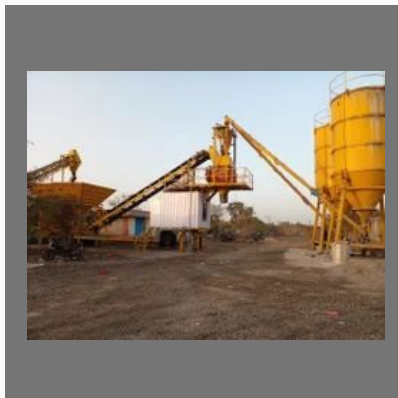
Rmc Ready Mix Concrete Plant
