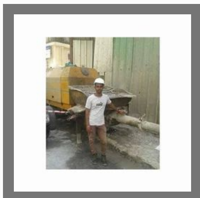
Concrete Pump On Rent
