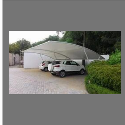
Tensile Car Parking Shed
