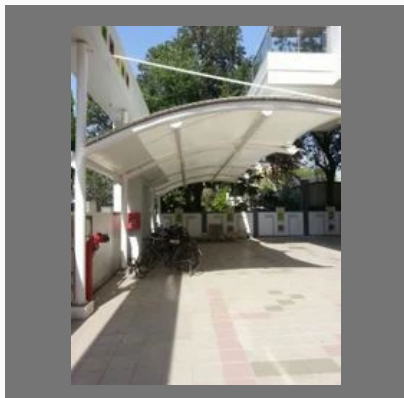
Tensile Membrane Structure Fabrication
