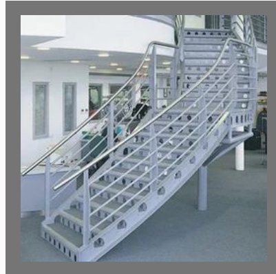
Mild Steel Staircase
