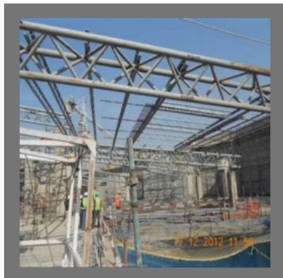
Skylight Structure Service
