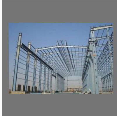
Pre Engineered Building
