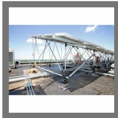
Solar Panel Support Structure
