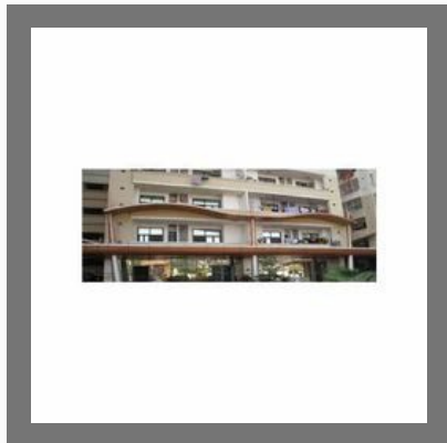
Main Entrance Canopy
