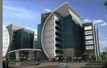
ACP Cladding And Toughened glass works
