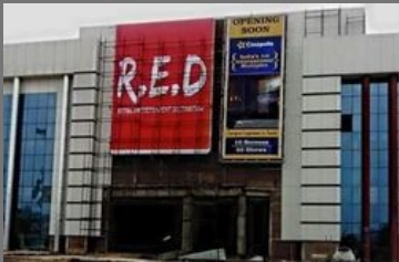
Aluminum Composite Panel Cladding
