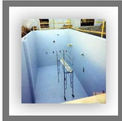
Tank Lining Service
