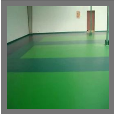
Epoxy & PU Floor Screeding
