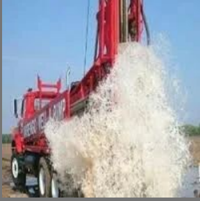
Drilling Bore Well Services
