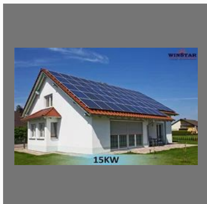
Solar Home Lighting System
