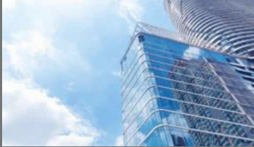
Glass Facade Glazing Service
