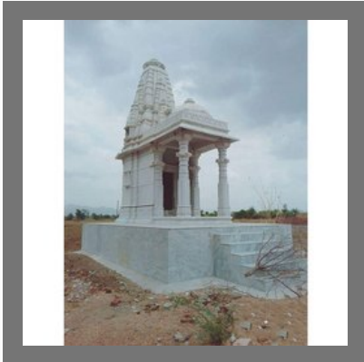
Temple Construction Service
