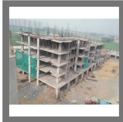
Residential Apartment Construction Service
