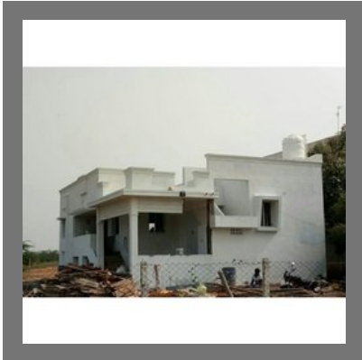
House Construction Service
