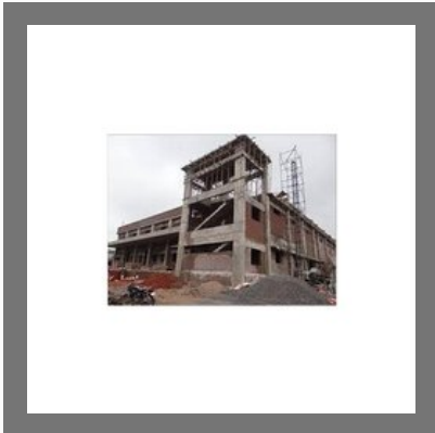
Commercial Building Construction Service
