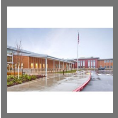
School Building Construction Services
