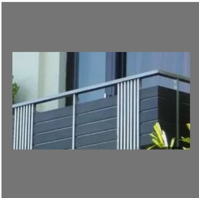
SS Balcony Railing
