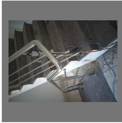
Stainless Steel Railing
