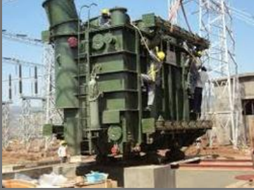
Erection & Commissioning of Transformers
