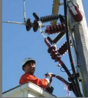
OH lines, Erection, commissioning, Operation and Maintenance
