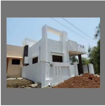
Residential Building Construction Work
