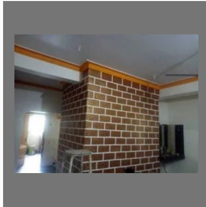
Residential Building Construction Work
