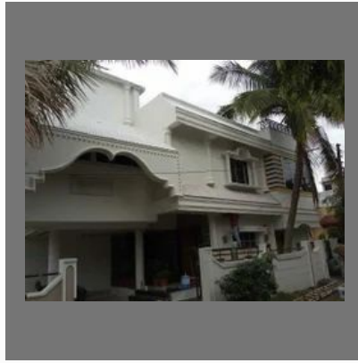
Residential Building Construction Work
