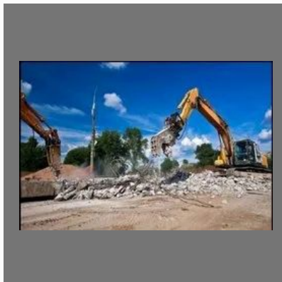
Building Demolition Contractors
