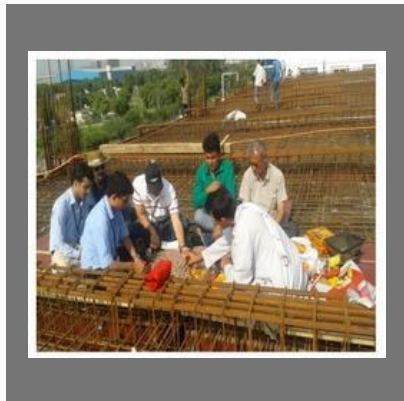
Commercial Building Construction Services
