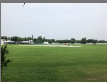
Cricket Ground Construction
