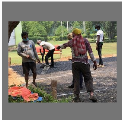
Society road construction
