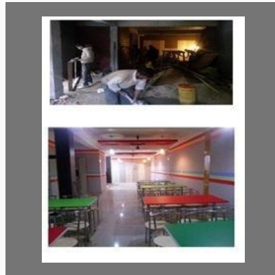
Cafeteria Construction Services
