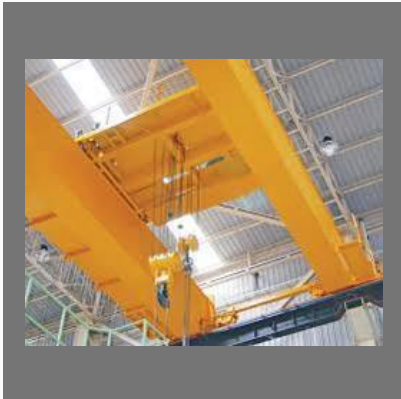
Eot Crane Cables
