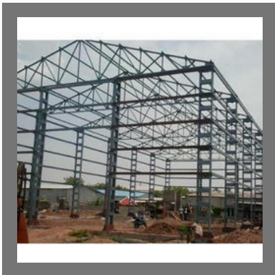
Structural Roof Fabrication Service
